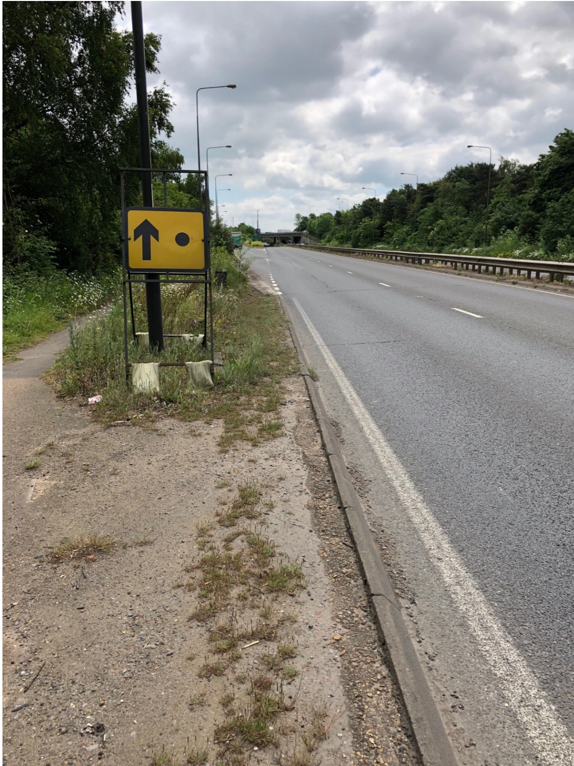
Photo 8.4.5: A23 Road Facing Southeast, 2019
